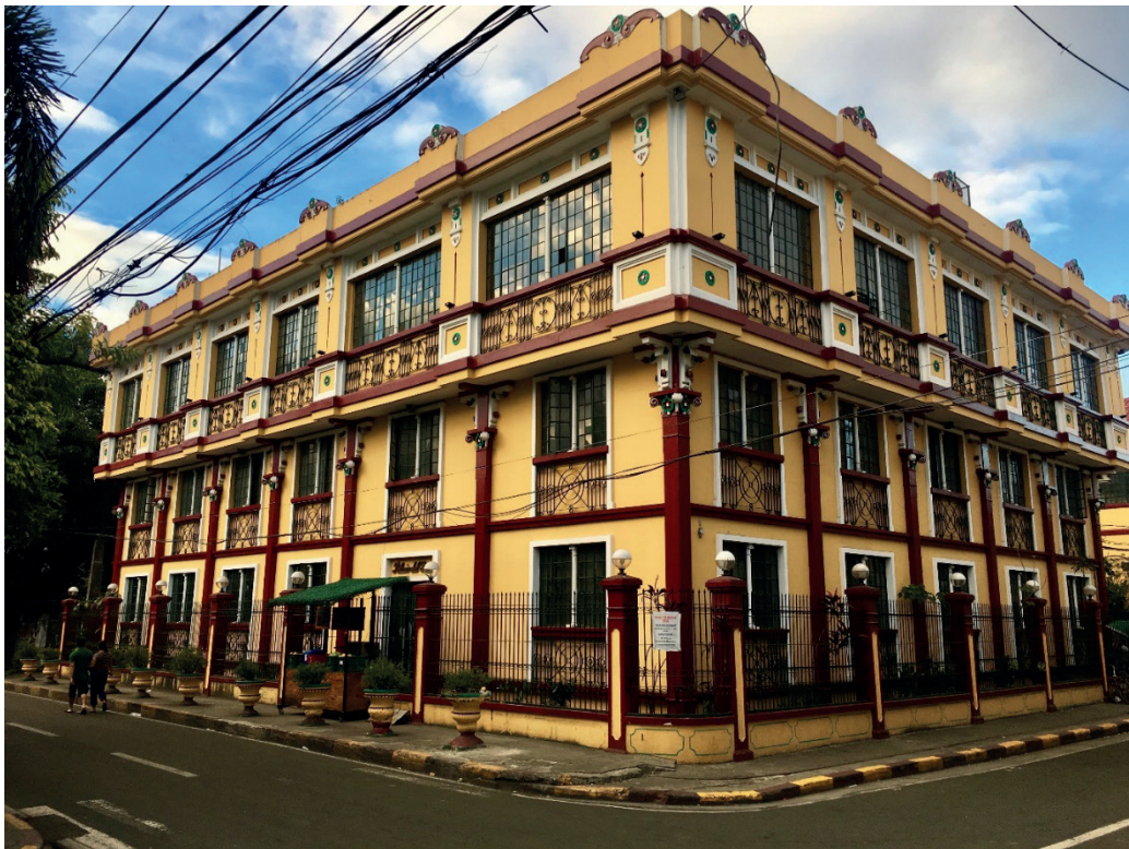
Photo 7: One of the buildings rehabilitated in Intramuros.
