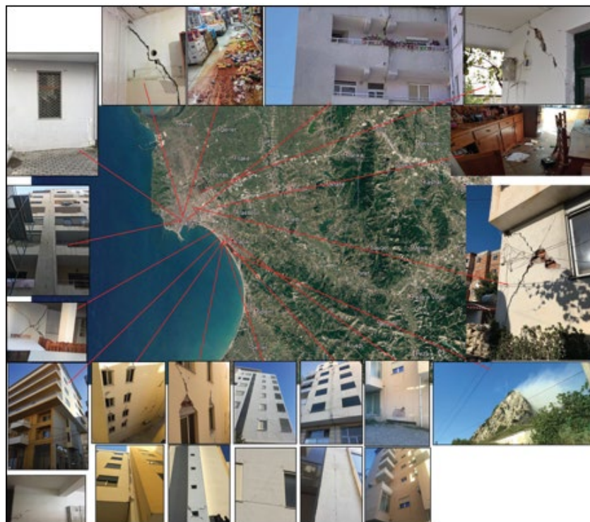
Figure 1. Photo of buildings damages in the epicentral area
