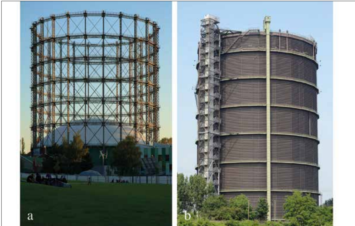
Fotoğraf 1a: Schöneberg Gazometresi su contalı teleskopik tipli gazometre, Berlin (Url 3). / Schöneberg Gasometer, a telescopic type gasometer with water seal, Berlin (Url 3).
