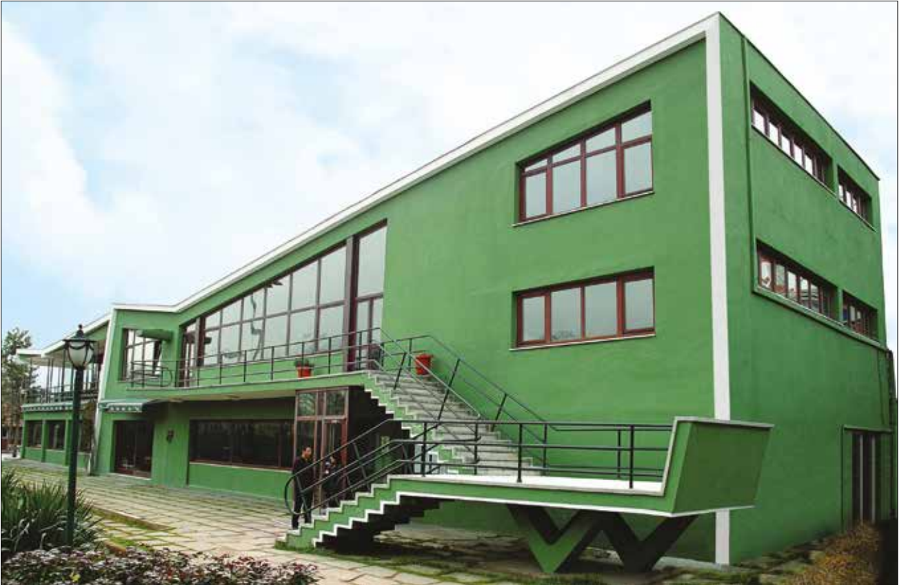
Figure 23 - Balcony and the staircase (TH&İDİL and TSMD Archive) / Balkon ve merdiven.
