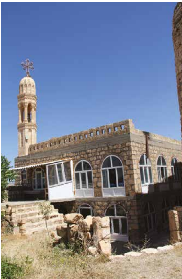
Figure 9 - New constructions in the village of Zāz / Zāz köyündeki yeni yapılar.
