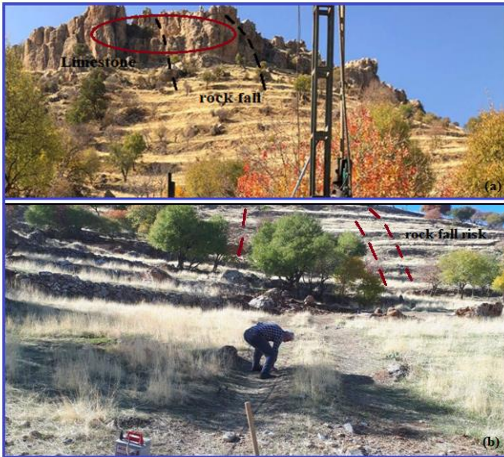
Figure 4. a) Close-up view and b) long-distance view of the study area
