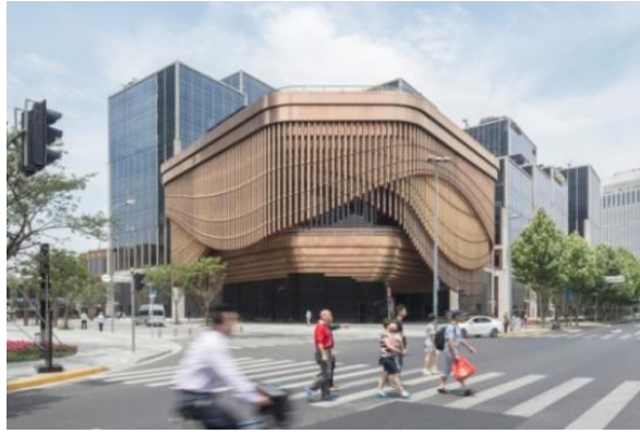
Şekil 27. Bund Finance Center (Archdaily, 2020c)
