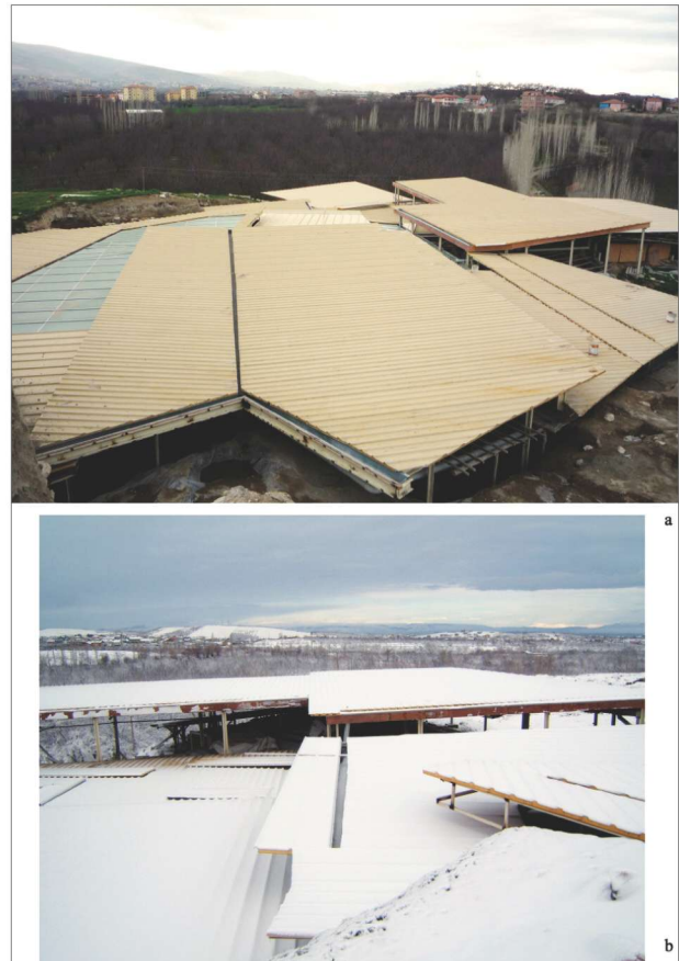
Fig. 4. Arslantepe, a: View of the roof on the 4th millennium palatial area from above; the different heights correspond to different building terraces. b: The roof under the snow in winter
