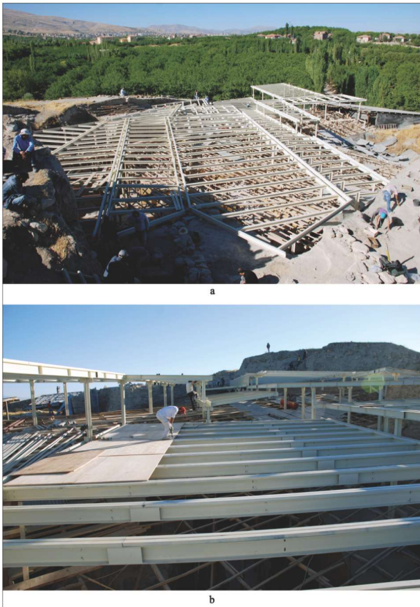
Fig. 3. Arslantepe, Horizontal metal structure of the roofing system
