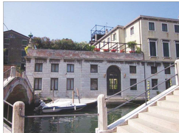
Fig. 12a. Palazzo Giustiniani, Water gate on Rio Ognissanti and altana (photo of the author)
