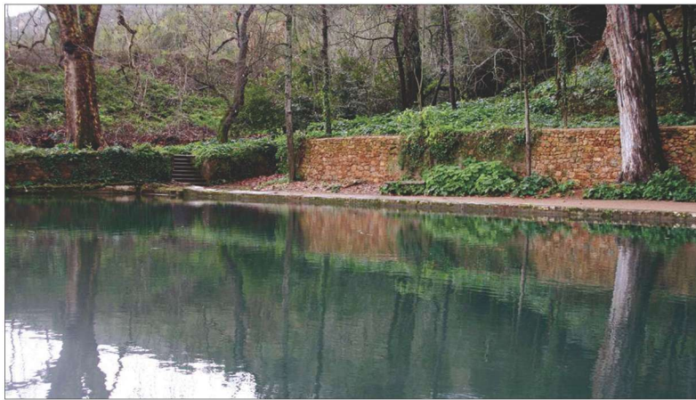
Fig. 7. Portugal, Quinta das Lágrimas, 17 th century tank storing water both for irrigation and powering the olive mill water wheel, 2006 (Antonio Sacchetti)
