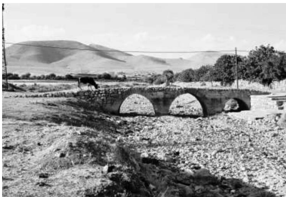
Photo 5. Harzem bridge in Kyzyltepa area of Mardin region
