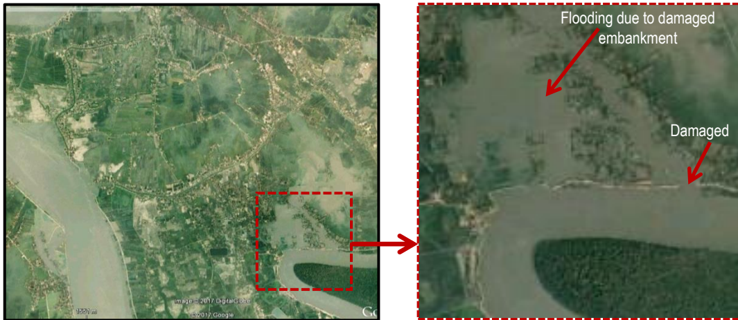
Figure 15: Worldview (Google) colour composite image of March 1, 2010 (Post Aila-2009) shows a small part of the present study: Damaged embankment allowing river water to spread up over the nearby land areas.
