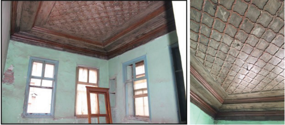
Fig. 26: Ceiling detail in site Z06 (By Karakuş, 2020)
