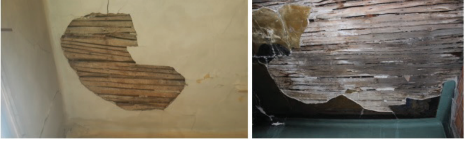
Fig. 22: Wooden piles in the ceiling of the sites 103 and 105. (By Karakuş, 2020)
