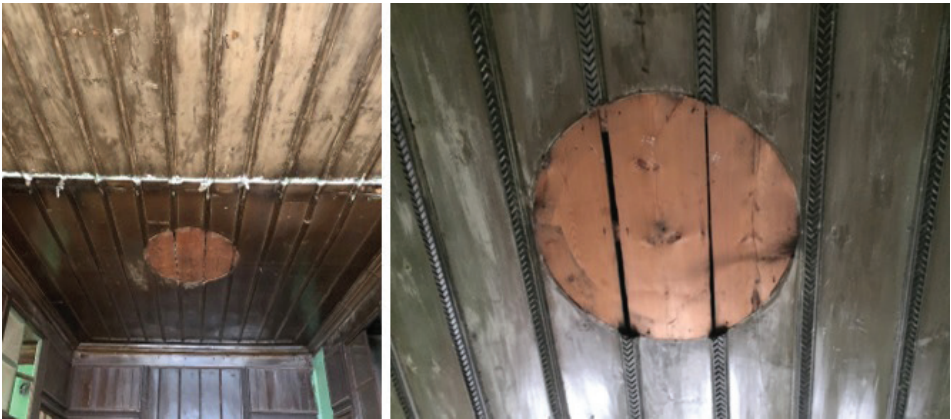
Fig. 23: Slatted wooden ceilings of the sites Z03 and Z05 and the location of the missing hubs. (By Karakuş, 2020)
