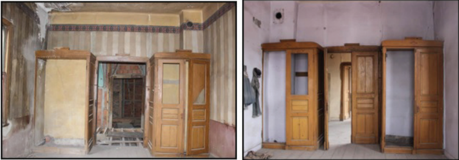
Fig. 29: Wooden closet and bathing cubicle in the sites no 106 and 108. (By Karakuş, 2020)
