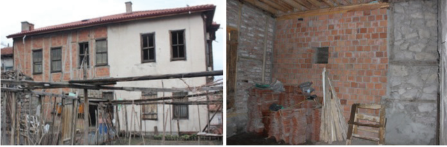
Fig. 18: Internal and external views of the renovated walls. (By Karakuş, 2020)
