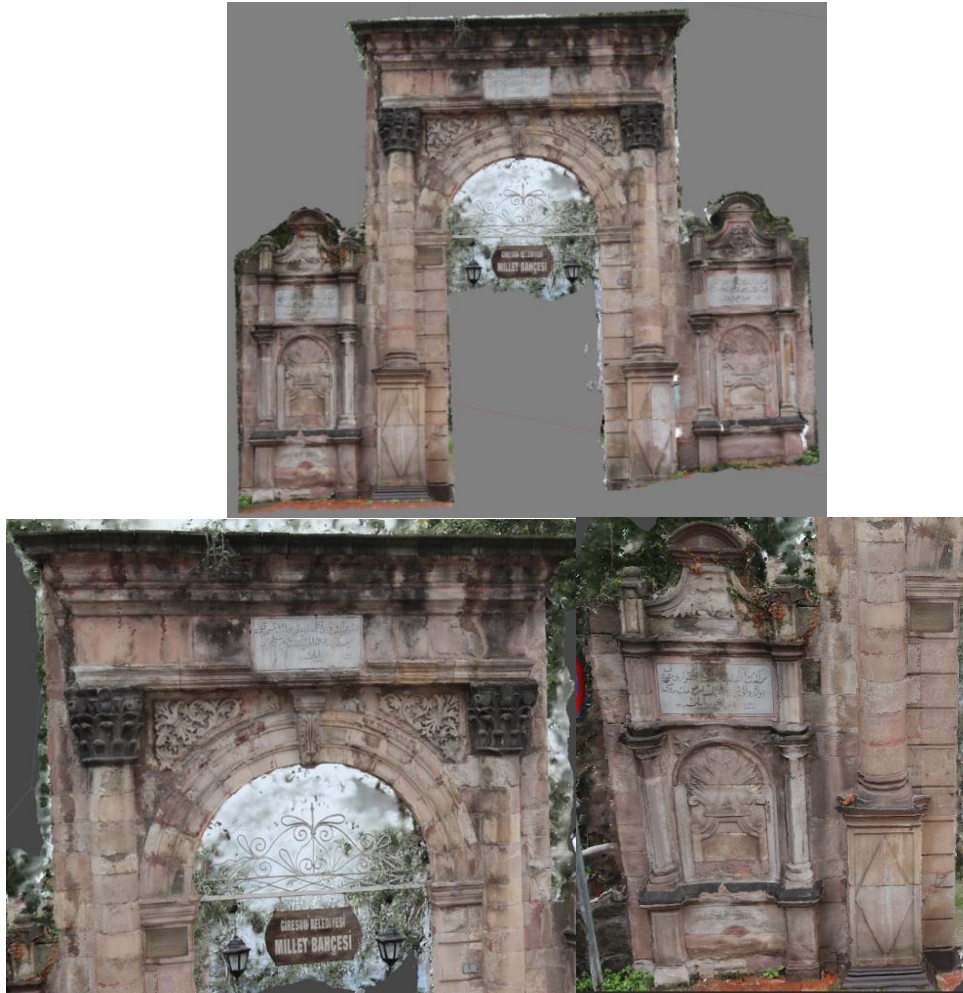
Figure 8: The 3D model view of the Public Garden door from different perspective
