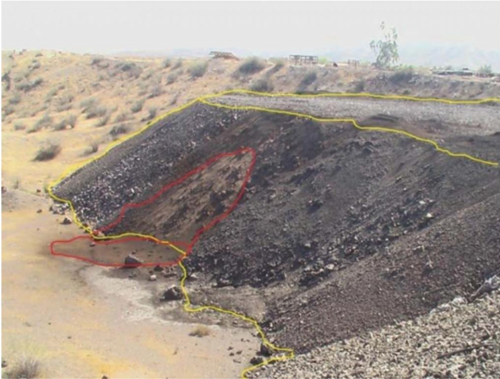
Figure 5. Discharge of refinery slag in valleys of mine region and occurrence of instability
