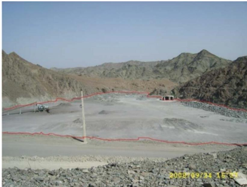
Figure 4. Waste discharge of underground mines in valleys of mine region and filling of them
