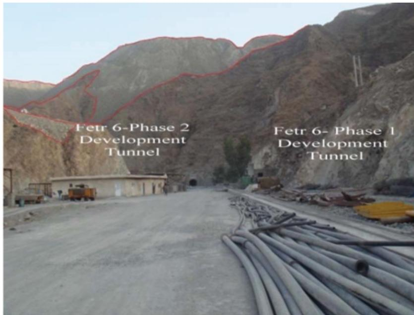
Figure 3. Waste discharge of surface mines above the phase 2 of Fetr6 underground mine
