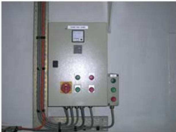
MOTOR STARTING PANEL
