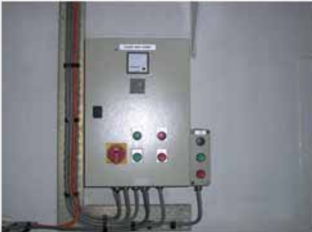
MOTOR STARTING PANEL
