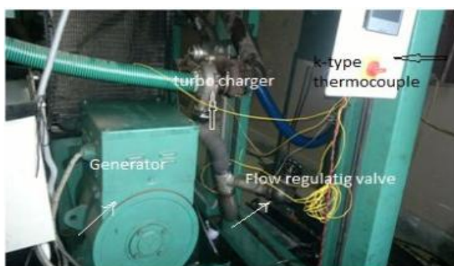
Figure 1. Photographic view of engine setup under turbo mode arrangement
