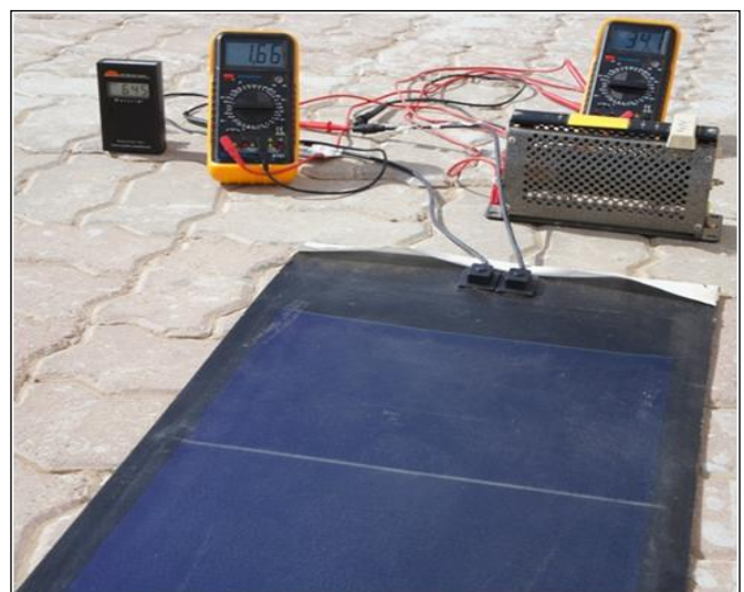
Fig.23. Setup of the PVL-124 solar laminate panel.
