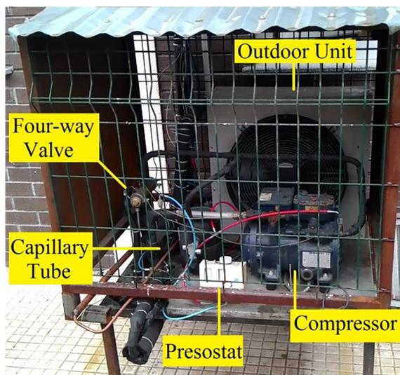
Figure 3. Outdoor unit of the heat pump
