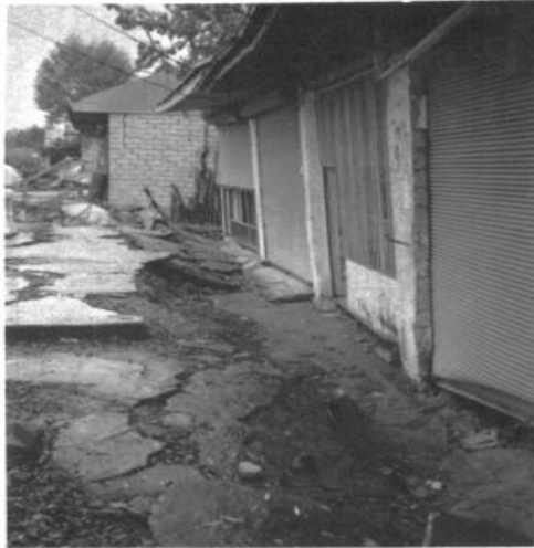
Figure 1. Liquefaction induced damages in Roudboneh, a town in the north part of Iran (Yegian et al., 1993).
