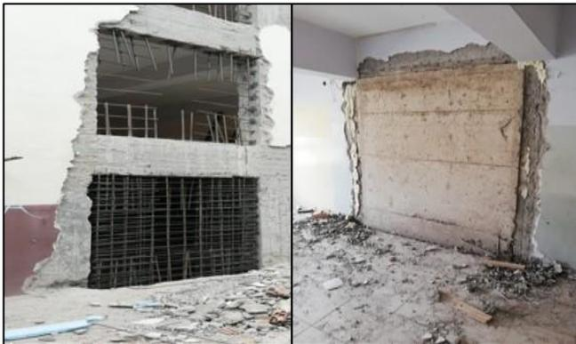
**Figure 4.** Adding shear walls
