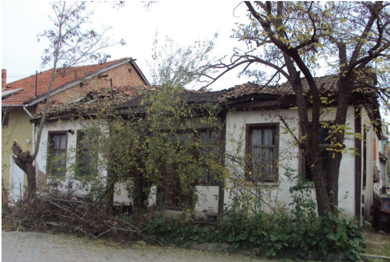
F. 13: Photograph Showing the Northwest Facade of the House (PA/18. 11. 2009)
