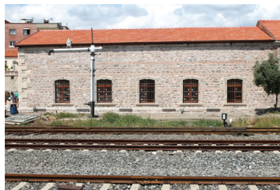
One of TCDD Hangar Buildings 59
