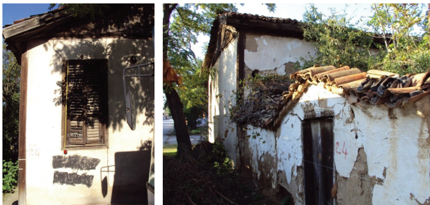
F. 17: Photographs showing the Southwest Facade of the House (PA/18.11.2009)
