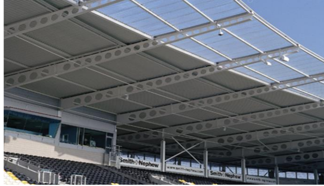
Figure 1: Roof support beams [18].
