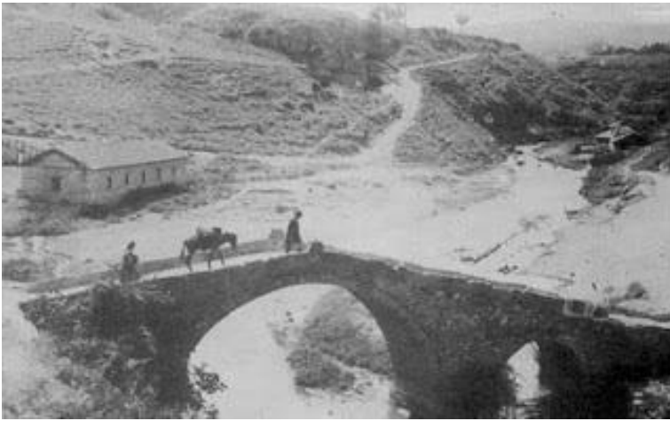
Figure 2. The bridge of Hatzikavoura in Veria. 19 th c. (Kalligas' archive)
