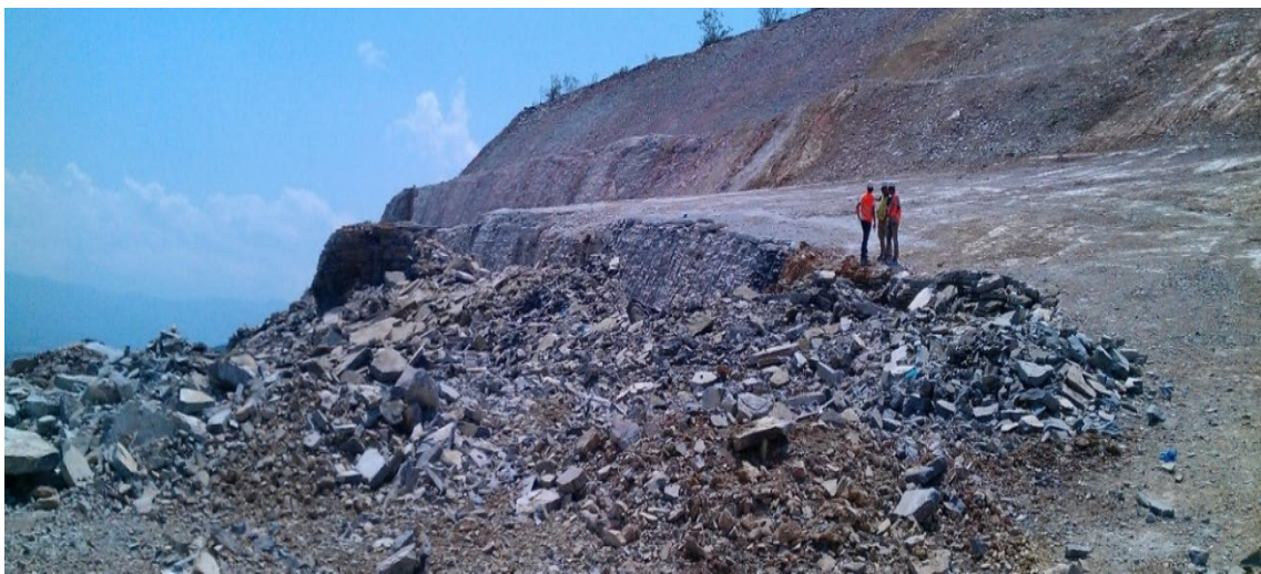
Figure 6. View from the results of contour blasting
