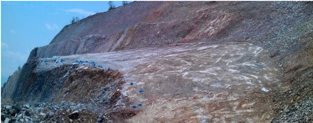
Figure 5. View of a case of contour blasting
