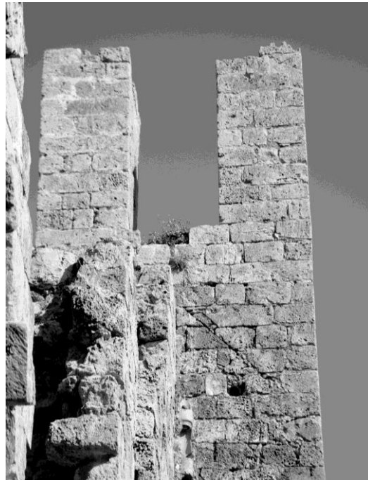
Figure 8. The added structure for hanging the bell on the buttress. Photograph by Hourakhsh Ahmad Nia.
