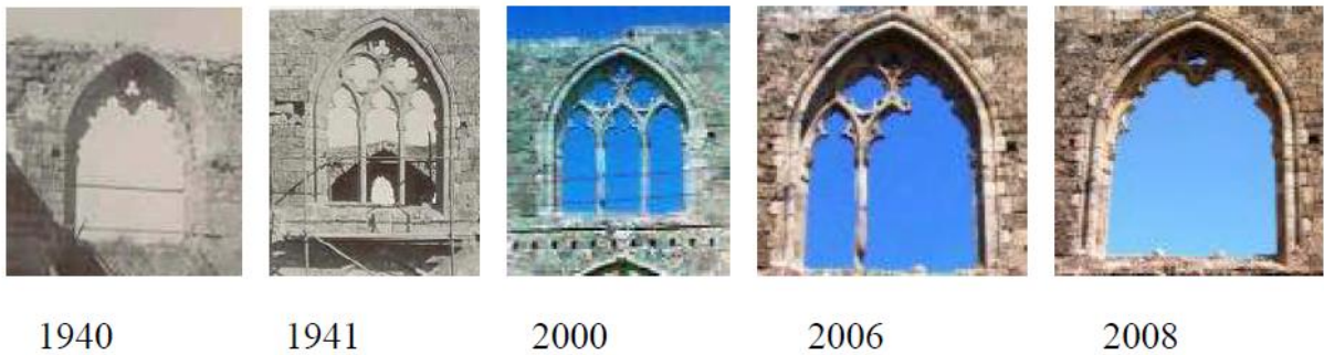
Figure 12. Window tracery above the main door [12].
