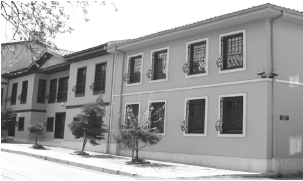
[a view of building on Kavaklı Street]
