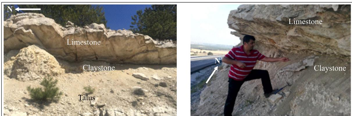
Figure 2- Thick limestone layers with a wide discontinuity spacing carrying the risk of rockfall due to undercutting processes of clay-bearing rocks (L7).
