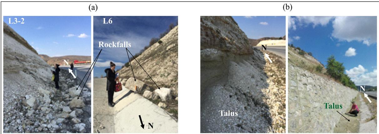
Figure 3- Geotechnical problems due to undercutting processes; a) rockfalls and b) the filling of road drainage ditches (Kütahya-- Eskişehir road, Ilıca location).
