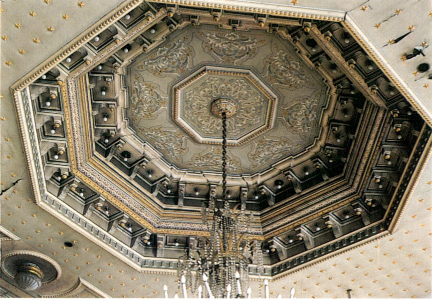
Res. 30 – Ahşap tavan - Merkezde yalancı kubbe. Wooden ceiling - Pseudo cupola at the center
