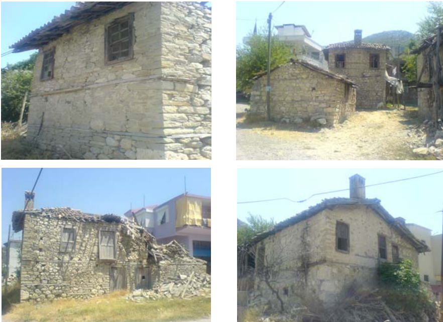
Fig. 2. Some examples for Turkish old masonry buildings (Original).
