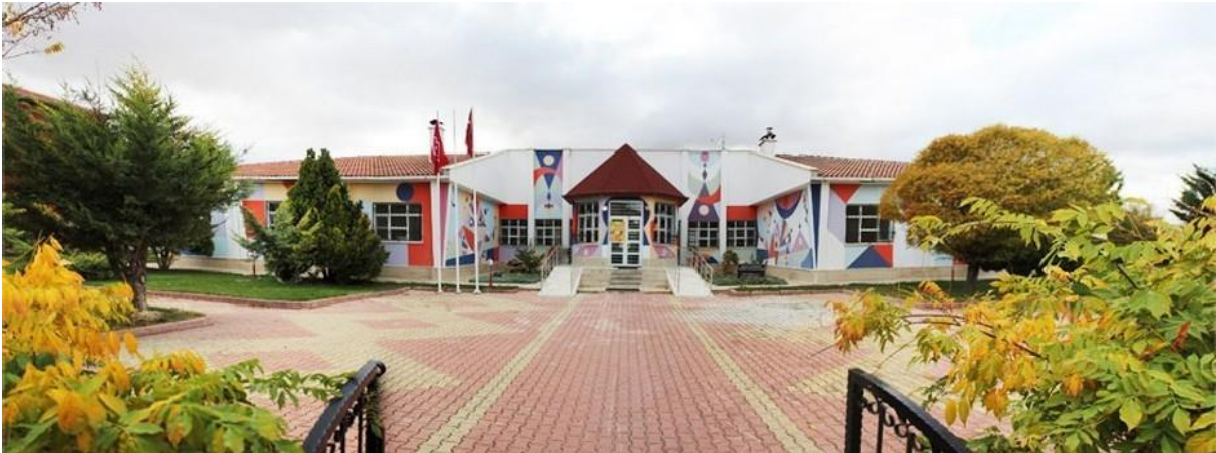
Figure 34. Back Yard Entry View
