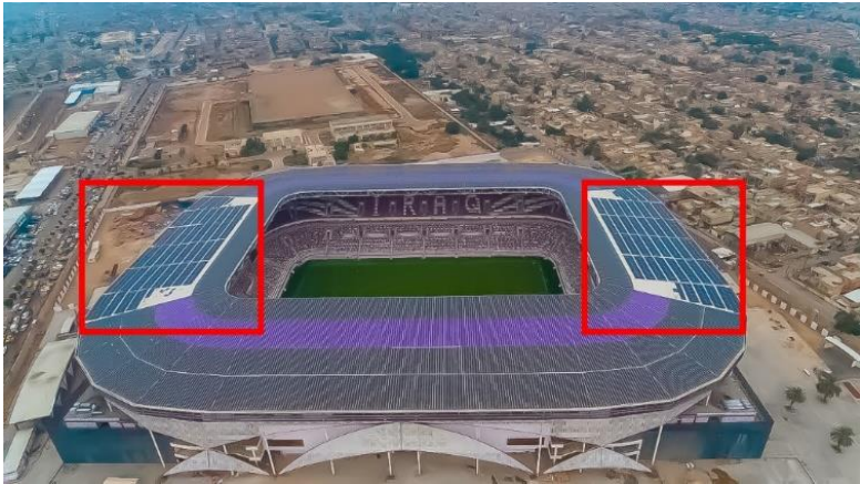
Figure 2 .Solar plates- International Shuadaa Stadium, Baghdad[11]
