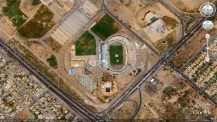
Figure 1. Stadium site and surrounding context. Source: (Google Earth)
