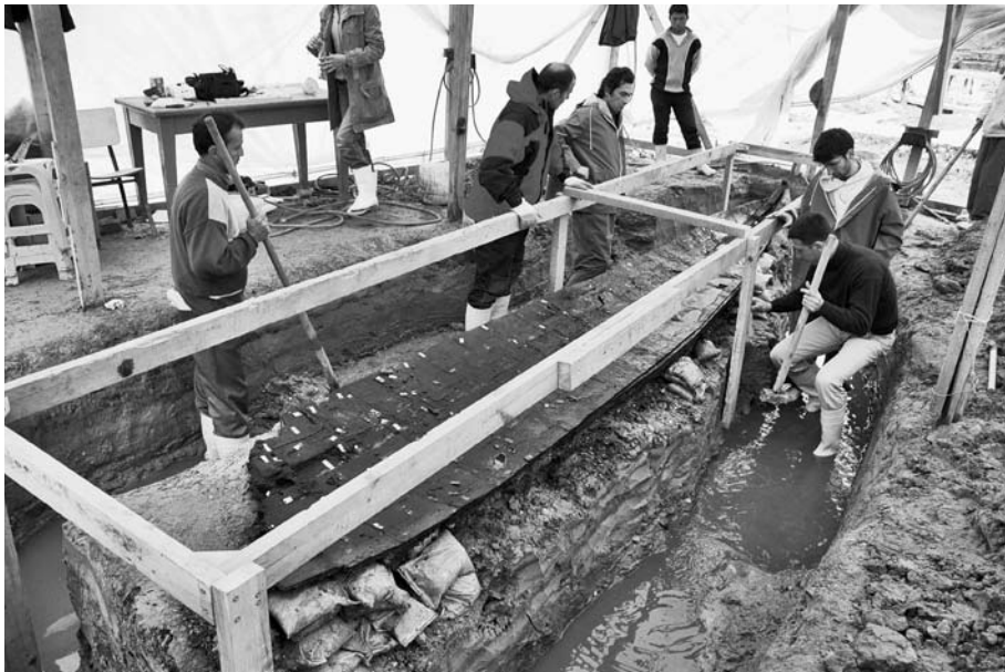
Fig. 6 Series of operations implemented from the beginning up to placing in the pool of the vessel in the method of lifting as a single mass (YK 6) (Photo: U. Kocabaş).
