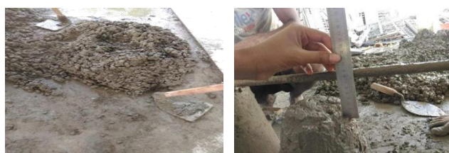
a). Mixing procedure b). Slump test Figure 2. Preparation of Concrete
