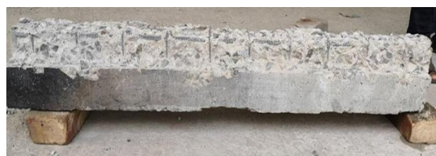
Figure 6. Chiseling of beam
