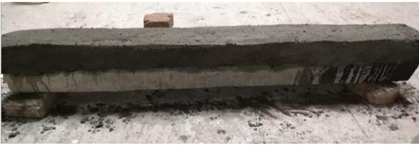
Figure 7. External strengthening of beam
