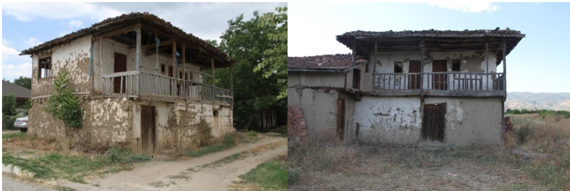
Figure 12. Examples of one and two-storey Alaçık around Tokat
