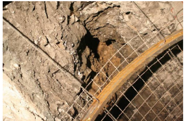
Şekil 14: Drenaj galerisinde güncel karstlaşma (km 0+253). Figure 14: Recent karstification in the drainage gallery (km 0+253).
