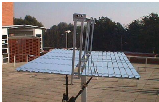
Figure 5. PV/T system at the University of Lleida terrace [25].
