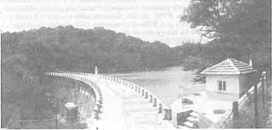
Resim 1 : II. Mahmut Bendi Figure 1 : Barrage de Mahmut II
