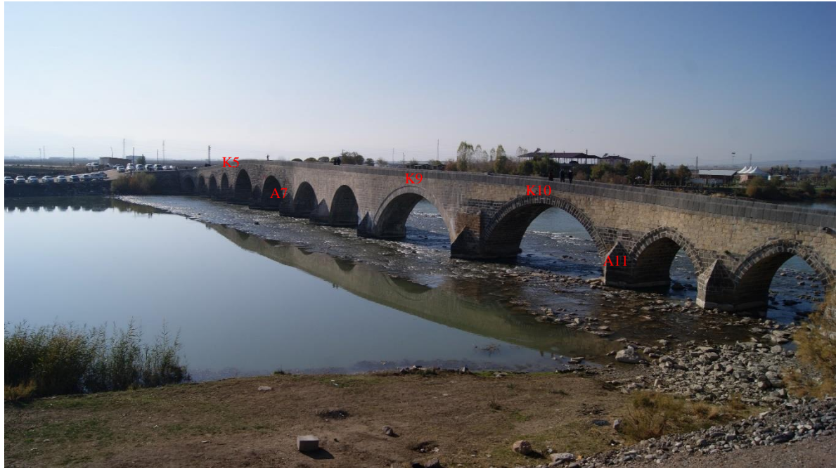
Figure 3. Historical Murat Bridge Upstream View (Present Condition November 2020)
