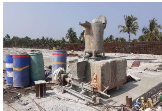
Figure 3. Single drum grouting mixer- Grouting equipment
