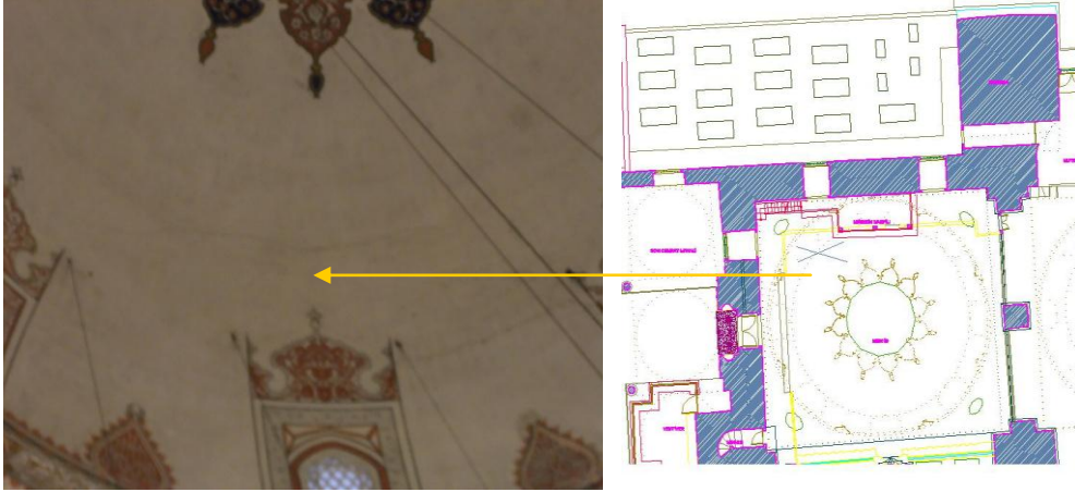
Şekil 17. Mescit kubbesinde oluşan çatlak ve plandaki durumu (Figure 17. The crack at the dome of the mosque and its projection on the plan)
