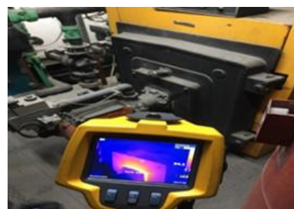
Fig. 7. Hot water boiler
