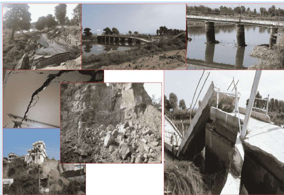
Fig. 2. Earthquake damages in around the epicenter in Jattalan Mir Pur City
