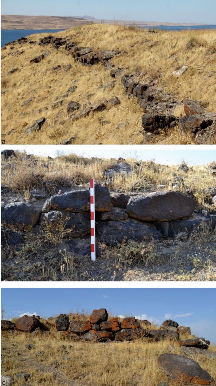
Fig. 5. Panz Fortress: (a) southeastern fortification walls, (b-c) detailed view of fortification walls, showing masonry and construction technique.
