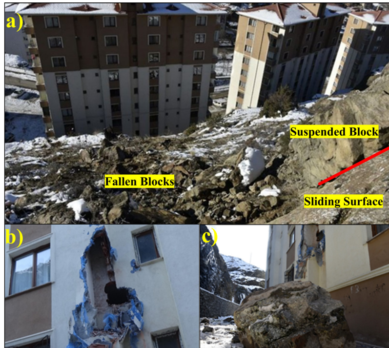
Figure 7- a) Oltanbey District Museum Houses Site. Andesite blocks that have broken off from the source rock areas (view direction from southeast to northwest), b) Oltanbey District Museum Houses Site. The building hit by the andesite block from the source rock areas (view direction from north to south), c) Oltanbey District Museum Houses Site. The building hit by the andesite block from the source rock areas (view direction from west to east).
