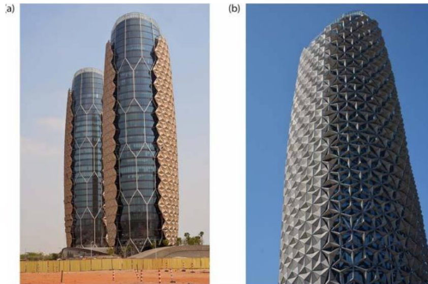
Figure 10. (a) Northern facade and (b) south facade of Al Bahr Towers, with some opened and closed shading devices [23]
