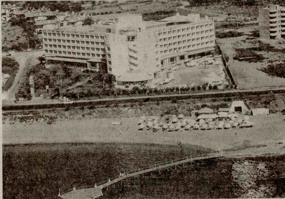
Foto 1- Alanya, Obaköy, Göl Mevkiinde 5 yıldızlı otel Photo 1- Five-Star hotel in Alanya, Obaköy, Göl Location
