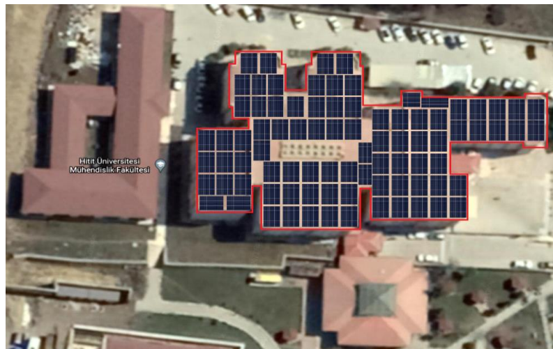
Figure 6. Hitit University Faculty of Engineering roof type solar energy system
