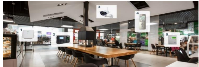
Fig. 4 Control systems inside a café
